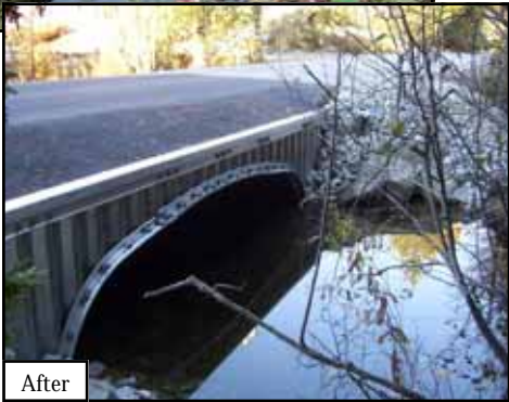
An open bottom culvert, bottom, replaced corrugated metal pipes, top, at Totten Road this past fall.
