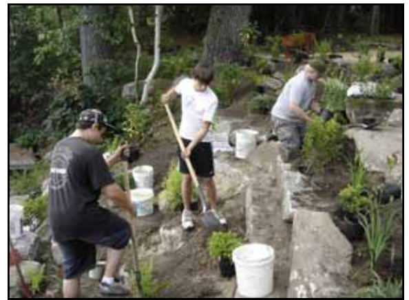
The Long Lake YCC installs a buffer for shoreline stabilization.
